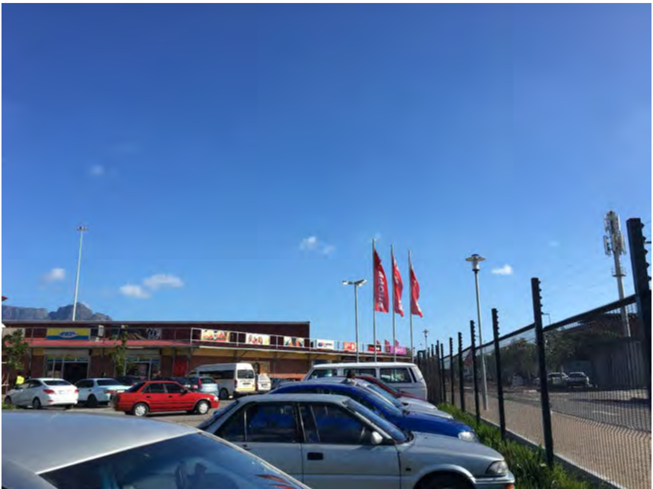
Figure 16: Langa Junction Mini Mall parking lot with the fence surrounding the Langa Junction Mini Mall (Source: Pulker, 2016)
