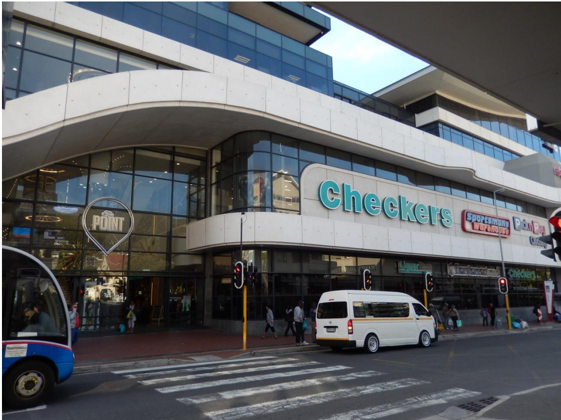
Figure 5-9 - The façade of The Point Centre which has Checkers as its anchor tenant (27 September, 2017).
