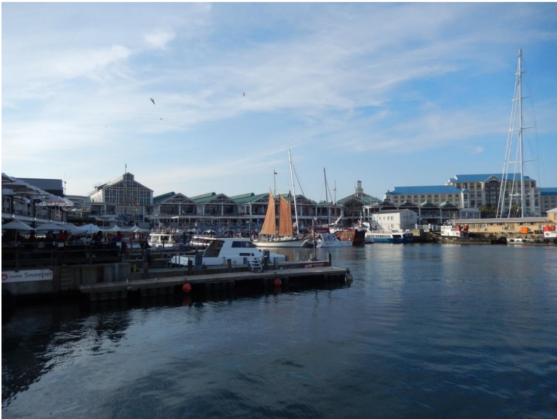
Figure 5-1 - The Victoria Wharf Shopping Centre at the V&A Waterfront development, Cape Town (24 September, 2017).
